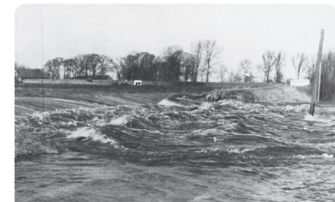
Sturmflut 1962, Deichbruch in Völlen
